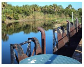
Pump Station 4 has 4 pumps (1 electric, 2 diesel, and 1 backup submersible) a telemetry system, and flap gates.
