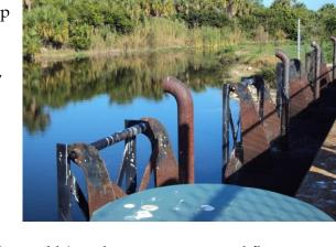
Pump Station 4 has 4 pumps (1 electric, 2 diesel, and 1 backup submersible) a telemetry system, and flap gates.
